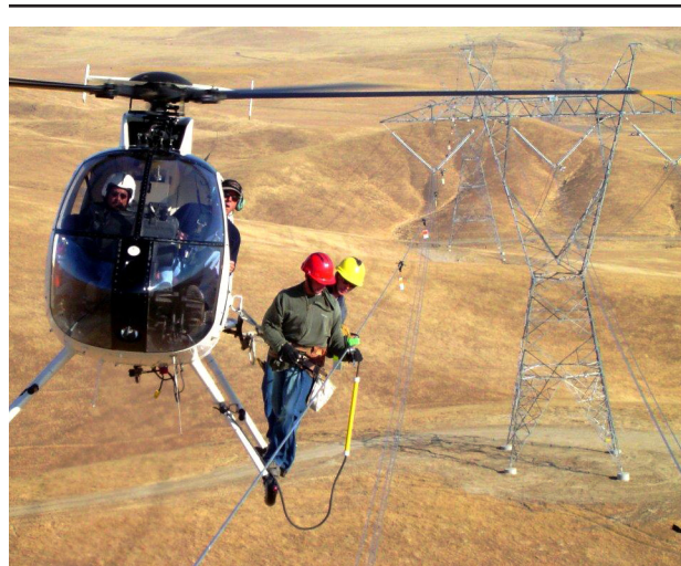
Installation by helicopter on existing power lines
